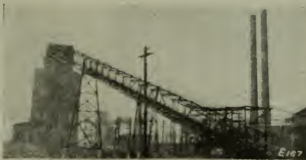
COKE QUENCHING PLANT DURING CONSTRUCTION.
